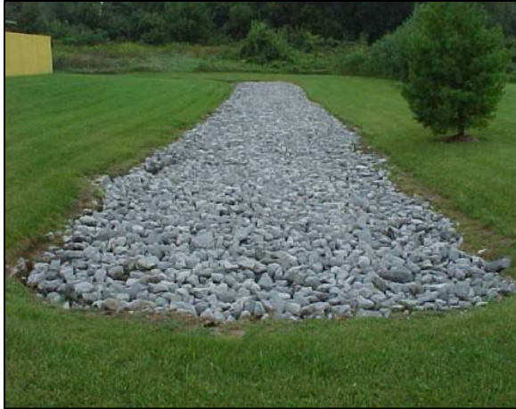
Image 6-7. Infiltration Trench. Source: AWWA. (2019, February 1). Infiltration trench: Do-it-yourself conservation practices. Acton Wakefield Watersheds Alliance. Retrieved October 7, 2021, from https://awwatersheds.org/infiltration-trench-do-it-yourself-conservation-practices/ .
