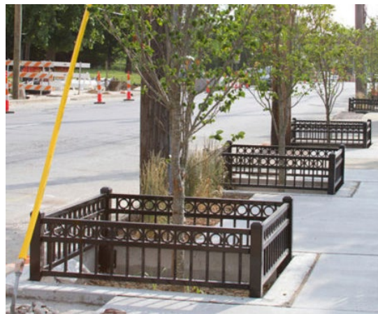
(Top) Image 6-4. A tree box installed with a speed bump to assist the flow of water towards the inlet. Source Photo: Pat Rector Rutgers, The State University of New Jersey, U.S. Department of Agriculture, and County Boards of Chosen Freeholders. Rutgers Cooperative Extension, a unit of the Rutgers New Jersey Agricultural Experiment Station, is an equal opportunity program provider and employer
