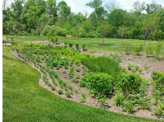
Image 6-2. Bioretention Systems Source: Bioretention System. New Jersey Future Green Infrastructure Developers Guide. (2020, May 7). Retrieved October 6, 2021, https://developersguide.njfuture.org/bmp/bioretention-system/ .
