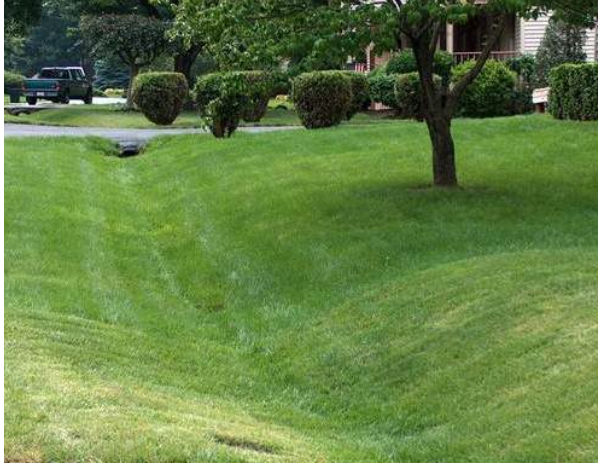
Image 5-6. Grassy channel. Source: Fairfax County Virginia. (n.d.). Control Heavy Runoff - Solving Drainage and Erosion Problems . Retrieved October 6, 2021, from https://www.fairfaxcounty.gov/soil-water-conservation/drainage-problem-control-runoff .
