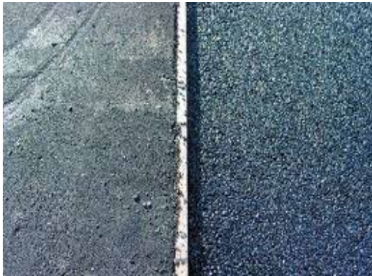
Image 6-9. Porous Asphalt. Source: Cornell University Urban Horticulture Institute. (2007). Using Porous Asphalt and CU-Structural Soil®. Retrieved October 7, 2021, from http://www.hort.cornell.edu/uhi/outreach/pdfs/cu_porous_asphalt.pdf .
