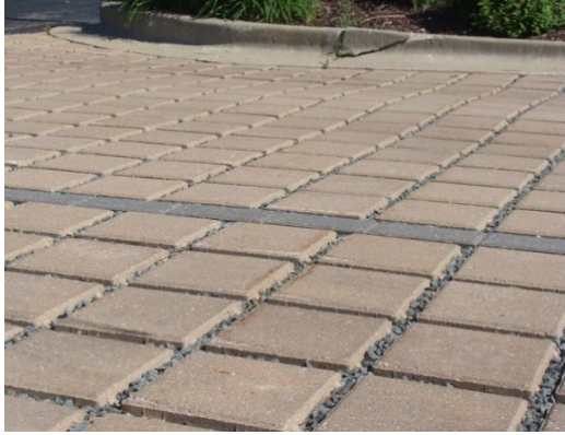
Image 6-8. Pervious Pavers. Source: Bay, A. for the C. (n.d.). Reduce your stormwater. Pervious Pavers. Retrieved October 7, 2021, from https://www.stormwater.allianceforthebay.org/take-action/installations/pervious-pavers .
